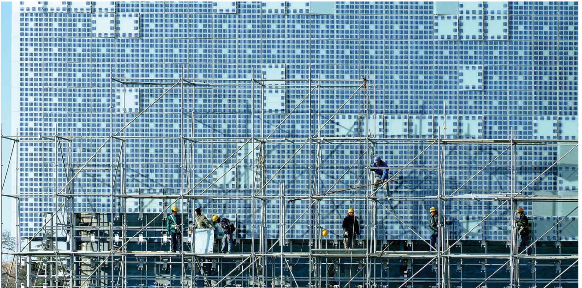
Installation of the Media Wall
