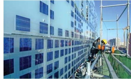
Workers on Site
