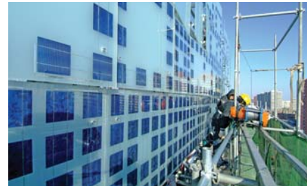
Workers on Site
