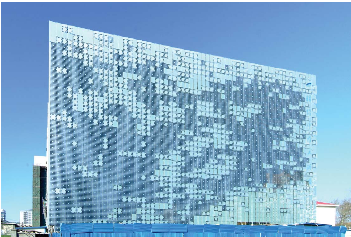
| The Media Wall During Construction
